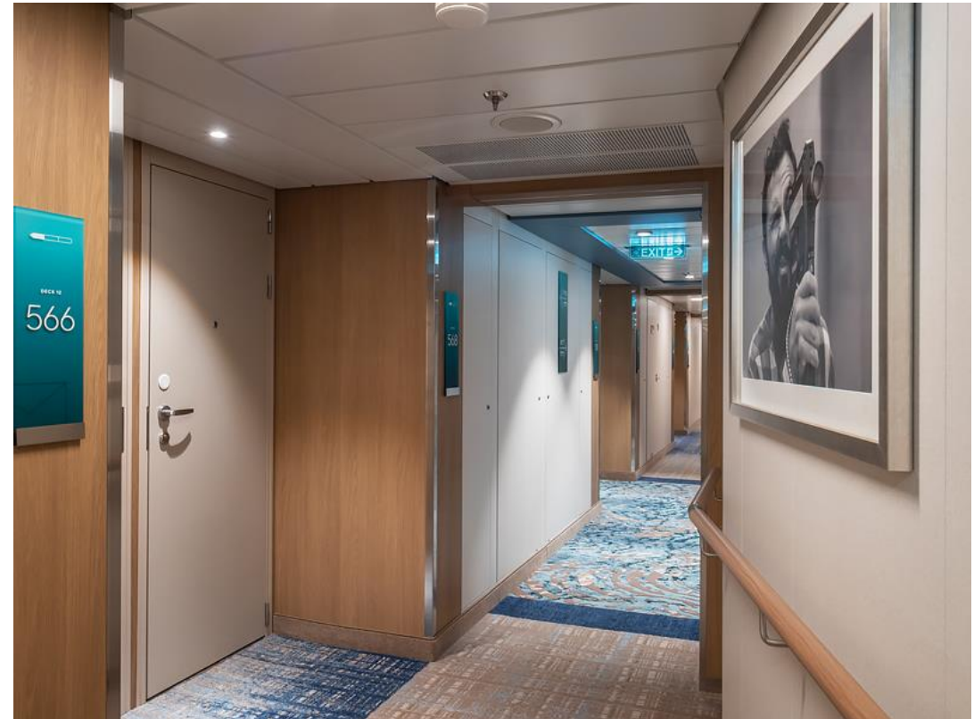
Lautex standard HT-300 B-15 ceiling on the vessel Icon of the Seas.
